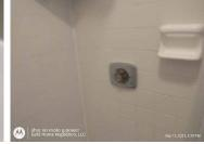
Shower/Surround: Tile - Noting crack across the shower floor. No visable leakage. This could leak into unit below.
