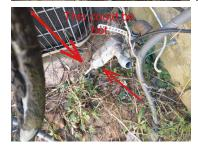
5. Main AC System Refrigerant Lines: Suction line and liquid line - Entry point not sealed
