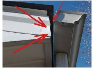
Downspouls. Noc. Downspouts: Noting smashed downspout in front driveway corner
