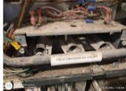
Blower Fan/Filter: Direct drive with reusable filter Gas supply line: Flex
